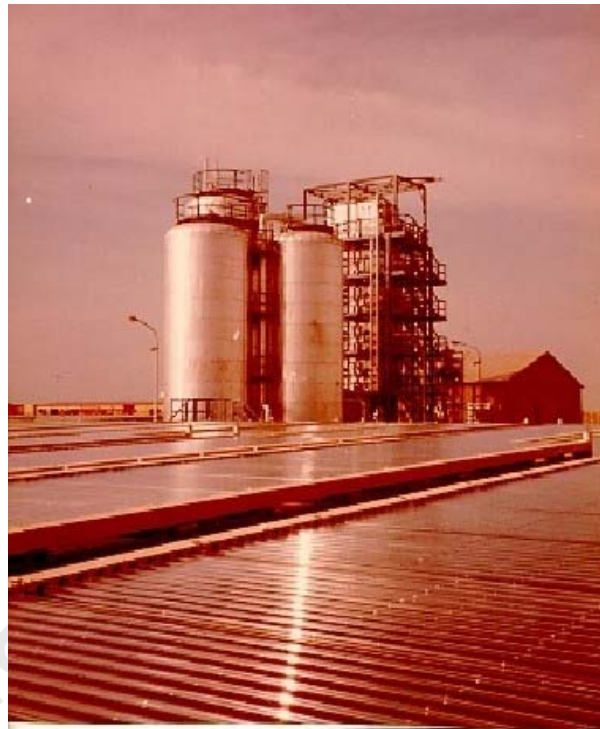
Figure 2. Photographic view of the solar desalination plant.
