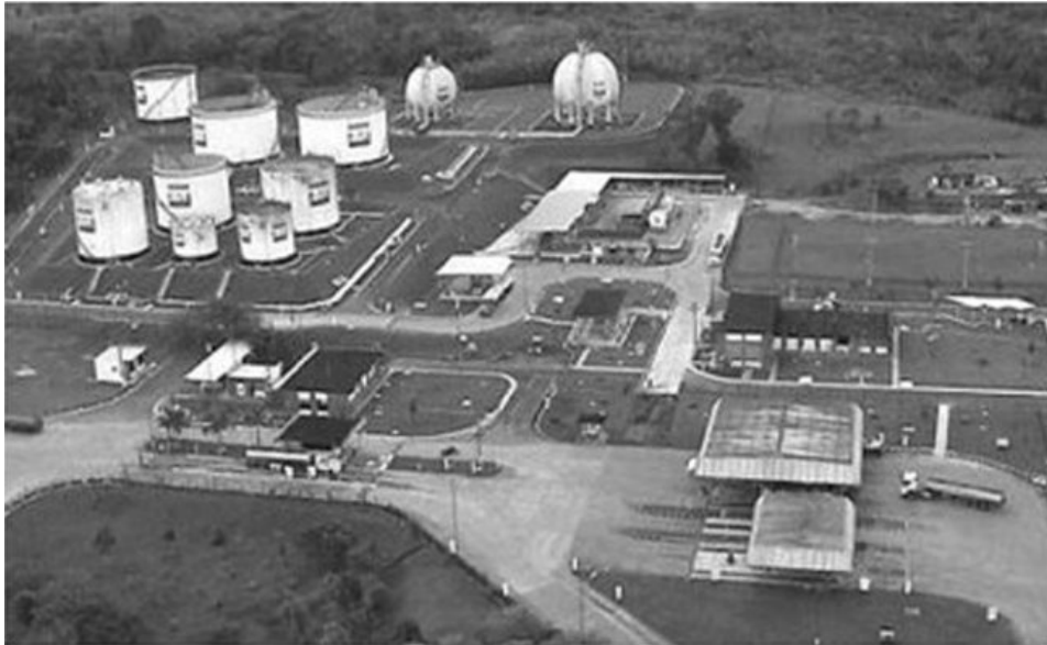
Figure 2 – An Example of a Pump Station
